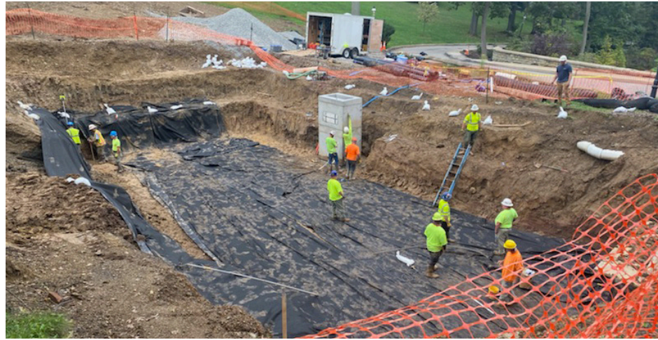
Underground construction is underway as the project team digs out a significant portion of Chapel Hill on Sept. 16. Photo Credit: Lilly Kubit
