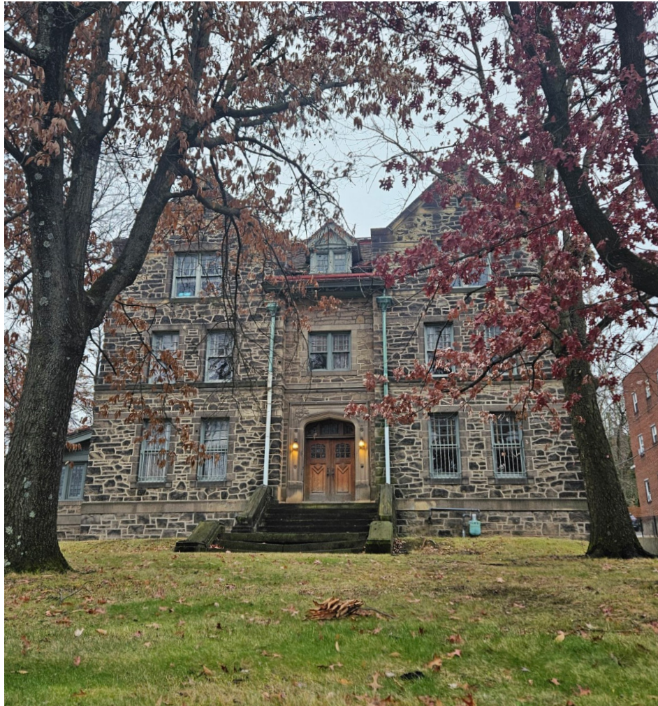
Outside the Thomson House located on Fifth Avenue. Sydney Altfather/Communique
